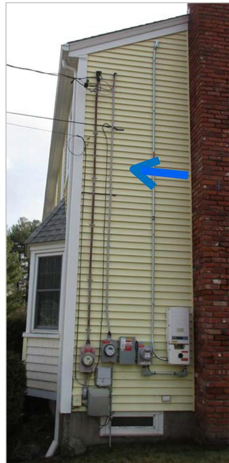
*Figure 4. New REG Electrical Service in Parallel with Existing Service*
